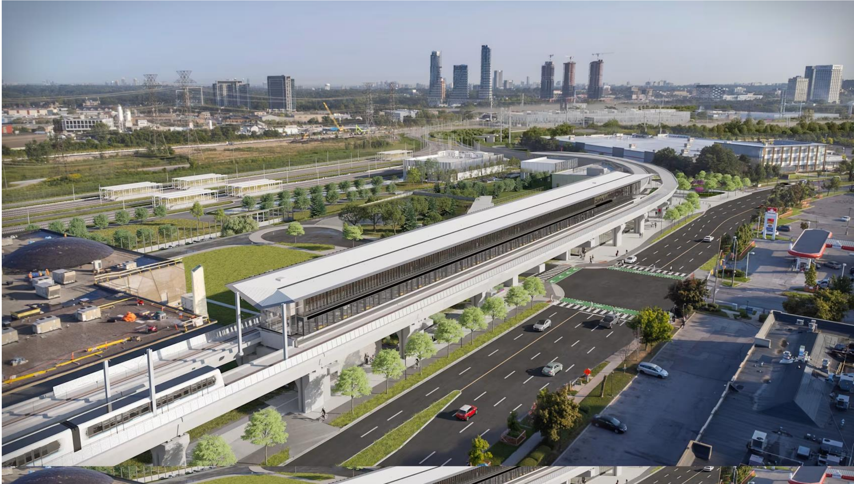
Future Ontario Line station at Thornccliffe Park, looking east from Overlea Boulevard.
